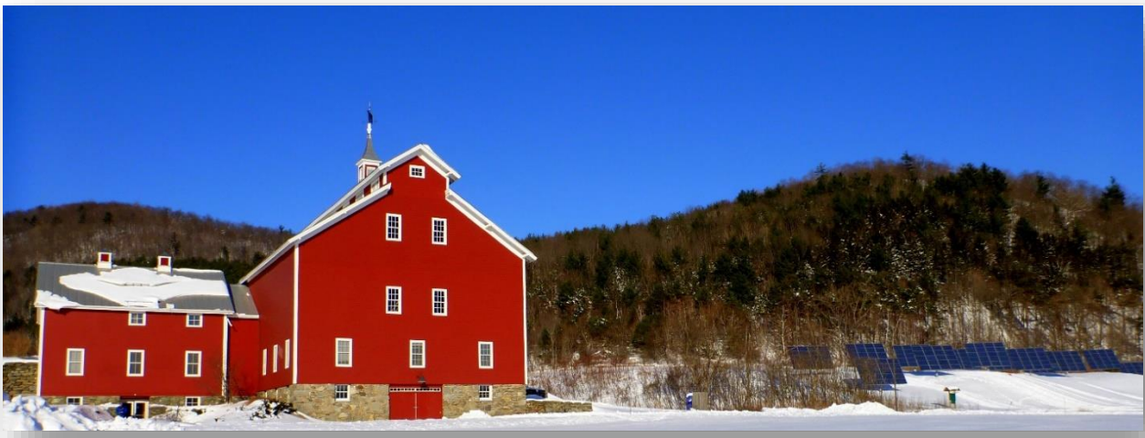
Figure 23 – VYCC Barn in Richmond – Source: CCRPC
